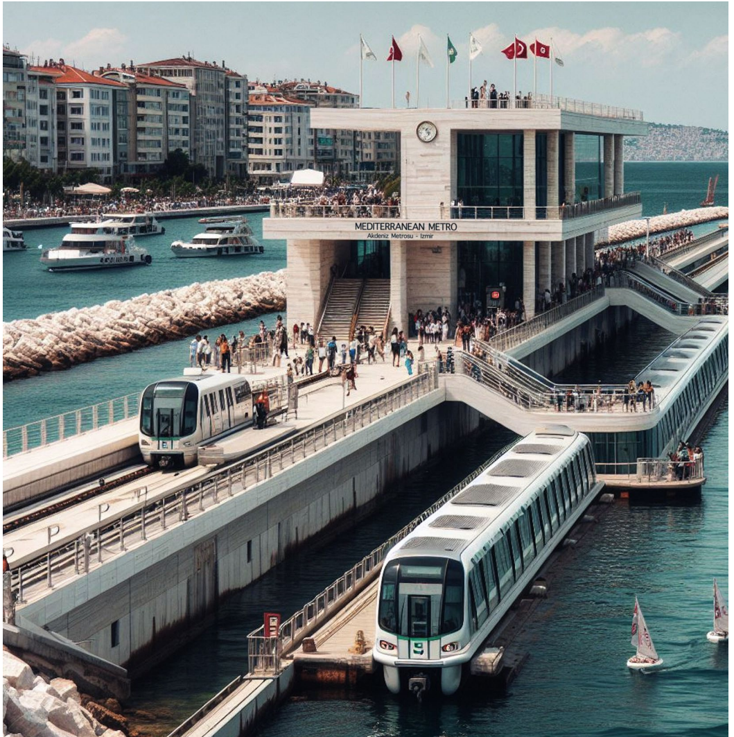
METRO STATION – IZMIR
