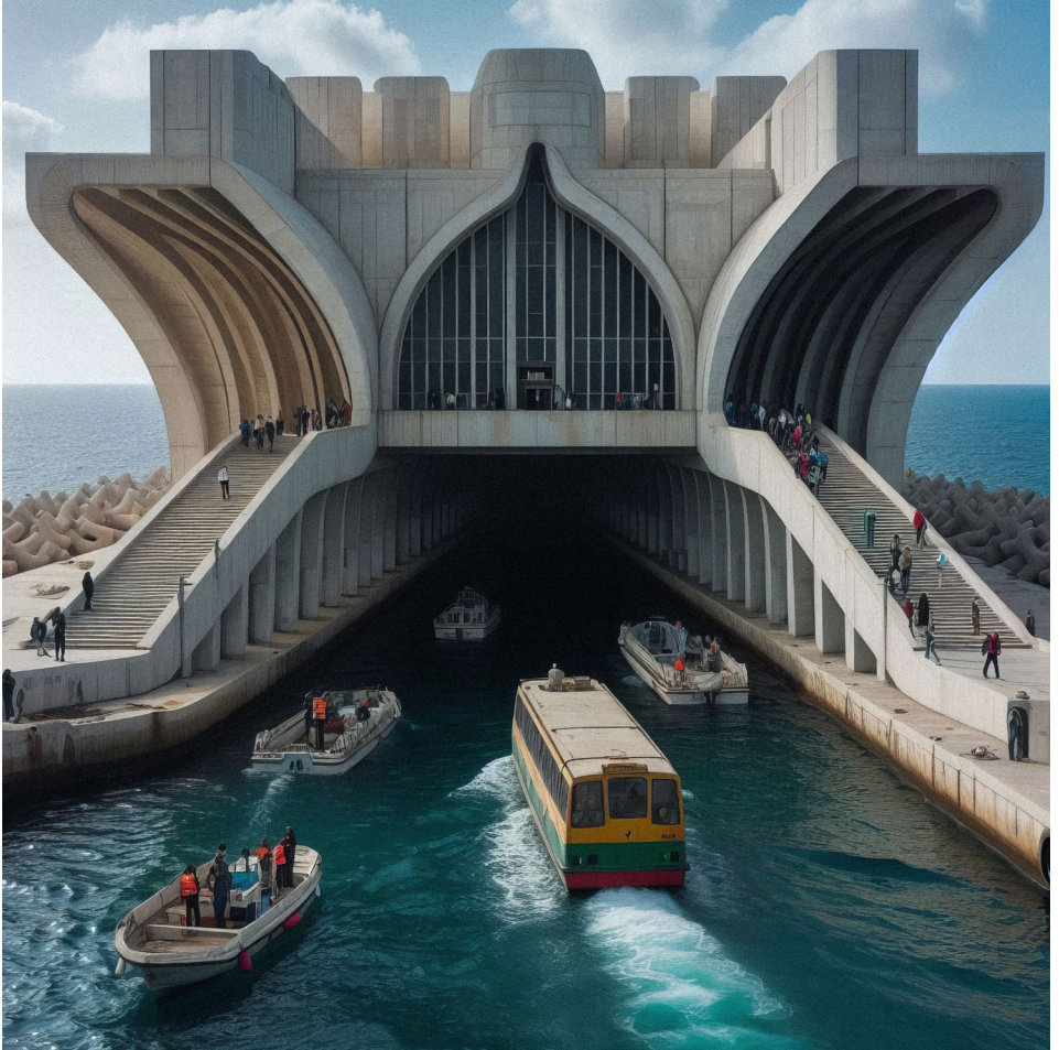
METRO STATION - TRIPOLI
